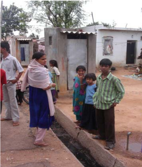
Drainage and latrines in Channapatna.
