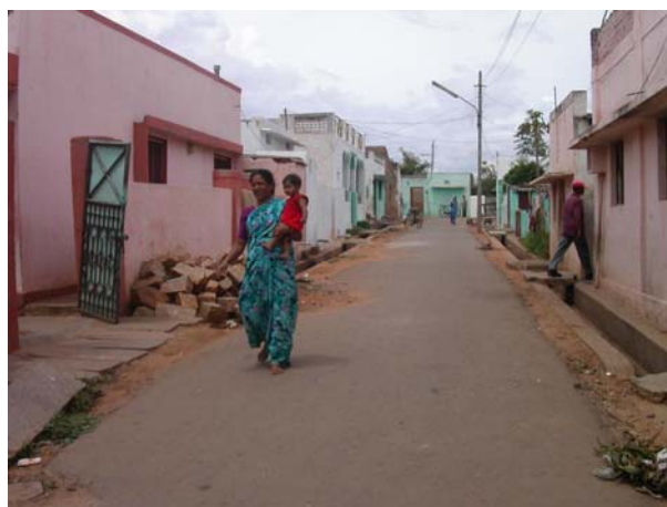
Improved road and drainage in Mysore.
