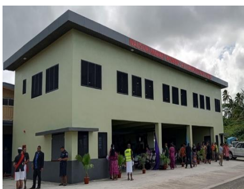
Nausori Market Rural Women's Accommodation centre, Fiji
