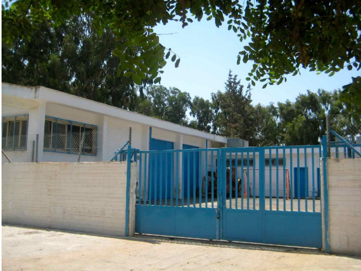
Picture 1: Renovated Diesel Agriculture Machinery Facilities at KTC
