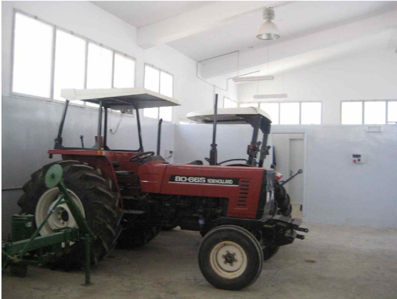
Picture 5 : Renovated Diesel Agriculture Machinery Facilities at KTC
