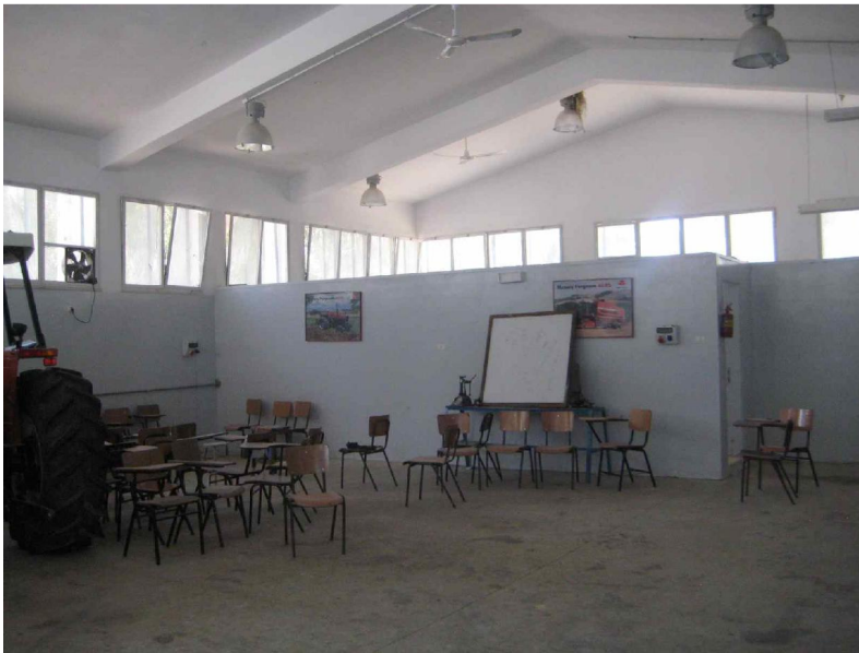
Picture 3 Renovated Diesel Agriculture Machinery Facilities at KTC
